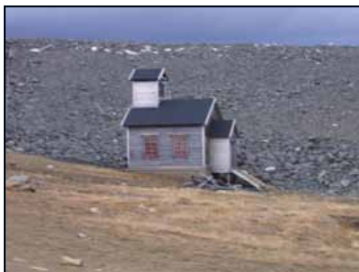
Trafo, Killingdal gruver, Holtålen
